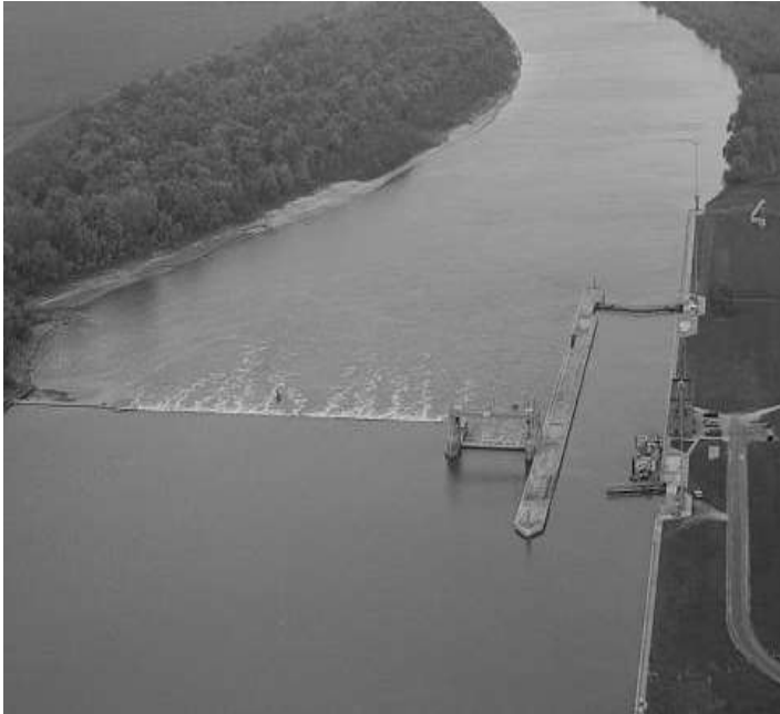
LaGrange Lock and Dam, Illinois River mi.80.2 (file photo)
